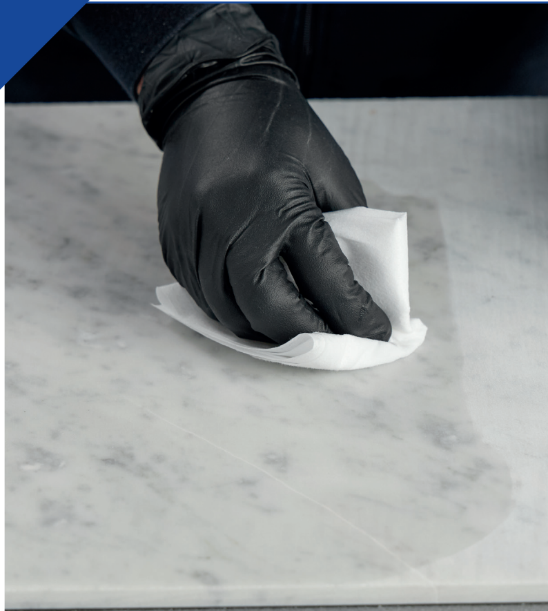
Apply the product to the back of the material to be laid
